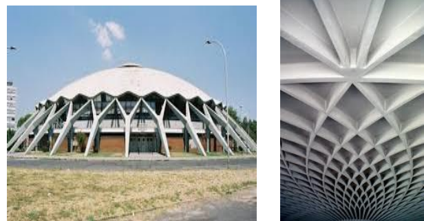
Fig 4: Sports Palace, Rome- structure and Ferrocement panels Source: Author
